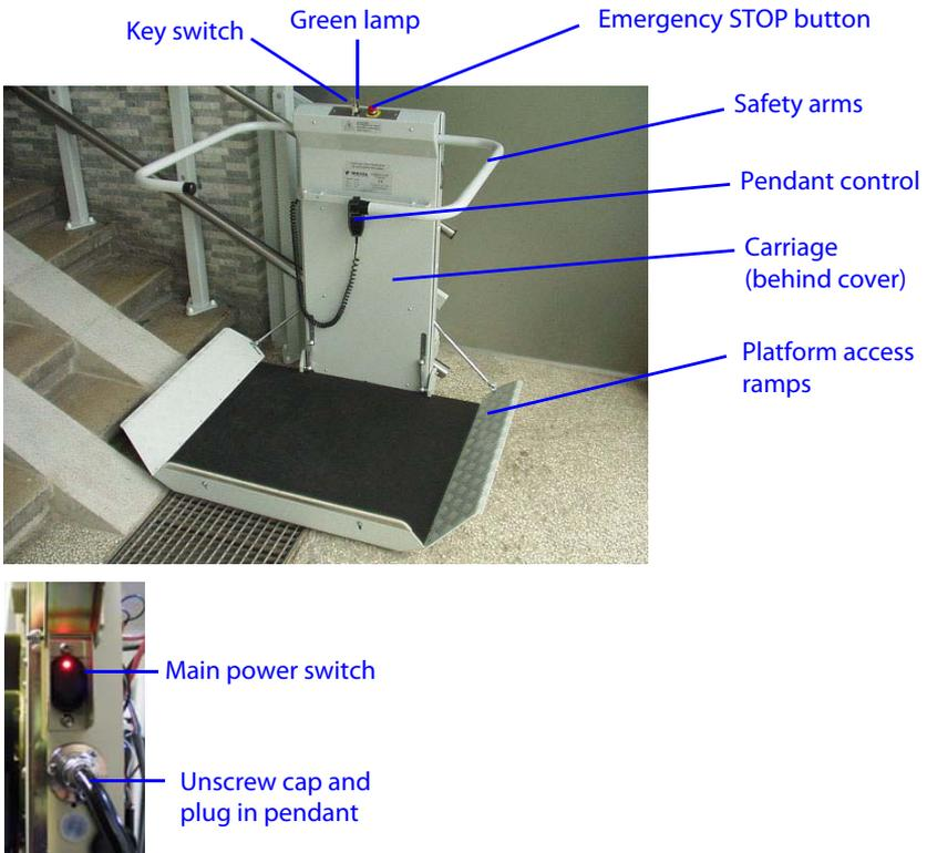
The drive unit (shown in Figure 2 below) has the following components:
